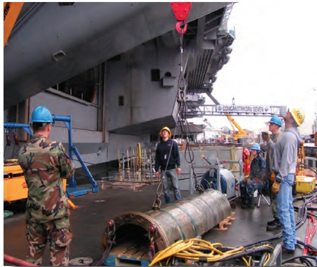
Alexander Grun and PSNSY Diver Dave Adams inspect the rigging as the crane prepares to lift the strut bearing shell off the support barge to divers waiting in the water.
